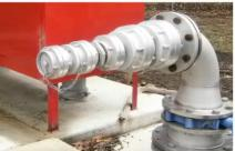
Figure 1: 150mm full bore isolation valve.
